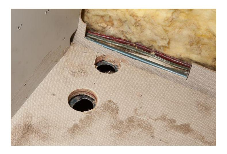
In order to enlarge the opening in the wooden floor, we take a scrap piece of 1x4" wood and drill a 2" diameter hole into it on your work table. Take this wooden template and center the 2" diameter hole over the hole you have already drilled into the cabinet floor. Temporary secure the scrap 1x4" piece of wood to the floor using two wood screws. Now place your 2" Hole Saw into the hole of the scrap 1x4" and proceed to enlarge the opening to 2" in the wooden floor ONLY
