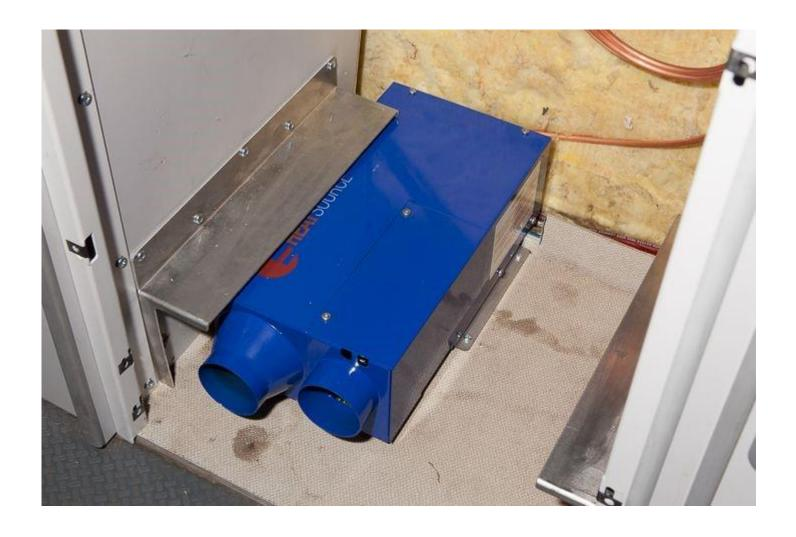
Place the **Vent Face Plate** in between the two **Side Support Mounting Plates.** This fitment should be pretty snug so be careful when placing it.
