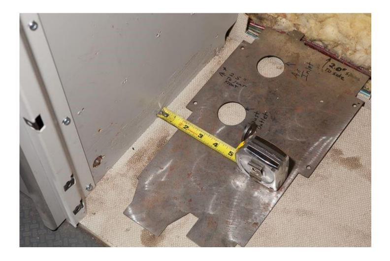
The back edge of the mounting ears on the template should overhang the edge of the wooden floor by 1/4".
