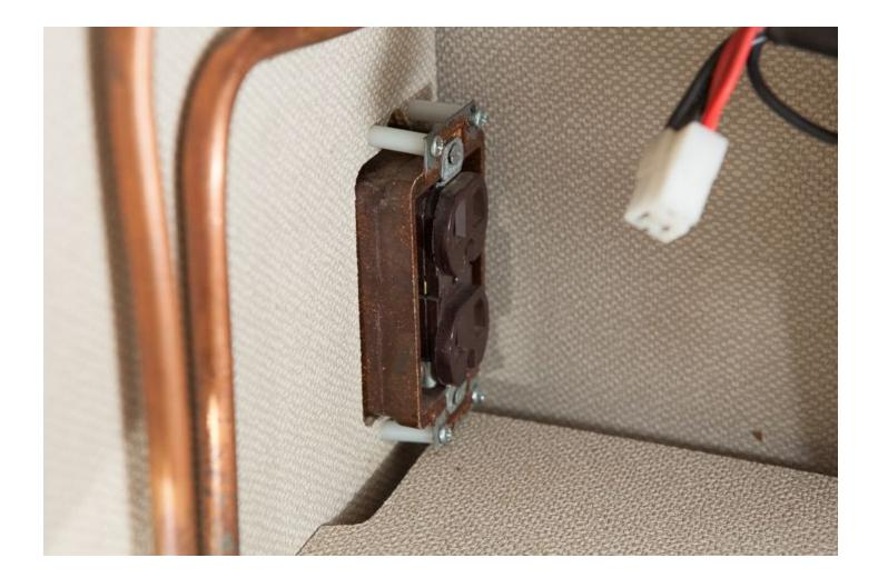
Use a **Small Flat Head Screwdriver** in order to reattach the AC Outlet faceplate back in place.
