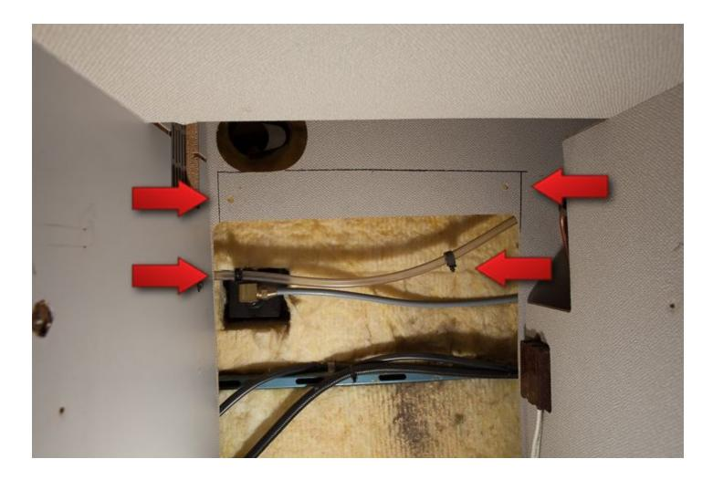
Use a **Small Flat Handsaw** in order to cut the fiberboard back wall out. Be very careful not to cut into the water line that we just freed from the fiberboard wall.
