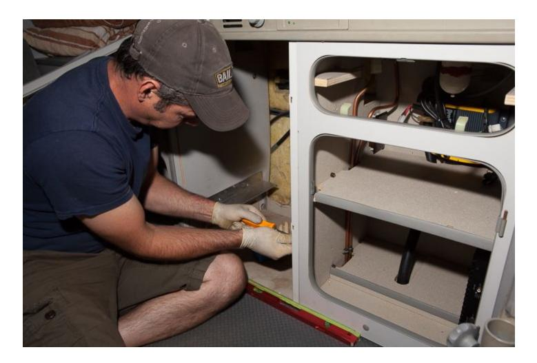
Place the left **Side Support Mounting Plate** into the fridge opening. Slide the **Side Support Mounting Plate** outward until the front of the **Side Support Mounting Plate** meets the backside of the level you're using as a guide.
