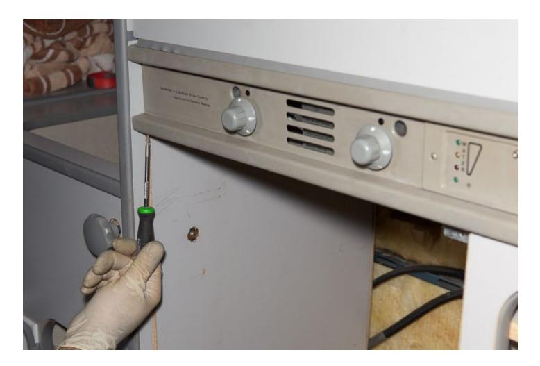
Use a **Phillips Head Screwdriver** to remove the bracket on the right side of the fridge opening. This bracket was used to mount the fridge surround to the cabinet. This is no longer needed and needs to be removed in order to not interfere with our kit.
