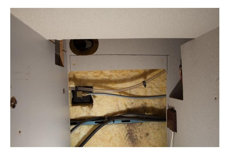
There are two clips holding a water line to the back side of the fiberboard wall that we need to remove. Press the clips back through the fiberboard so that they're clear and place the water line down low below the area we need to remove.
