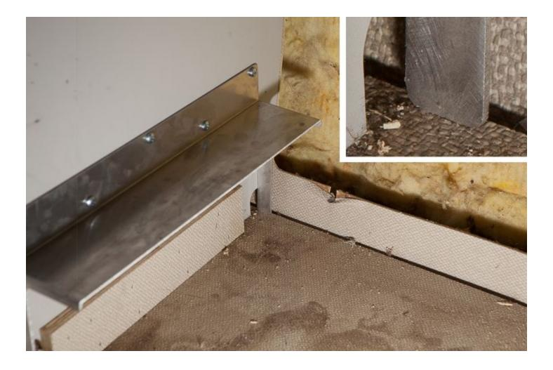
Repeat the process for the **Support Bracket** on the right side of the fridge opening. In our case you'll notice we can't locate the vertical leg of the **Support Bracket** far enough to the rear so it's flush with the edge of the cabinet floor. The small section of wood stapled to the wall is too far forward to allow it.
