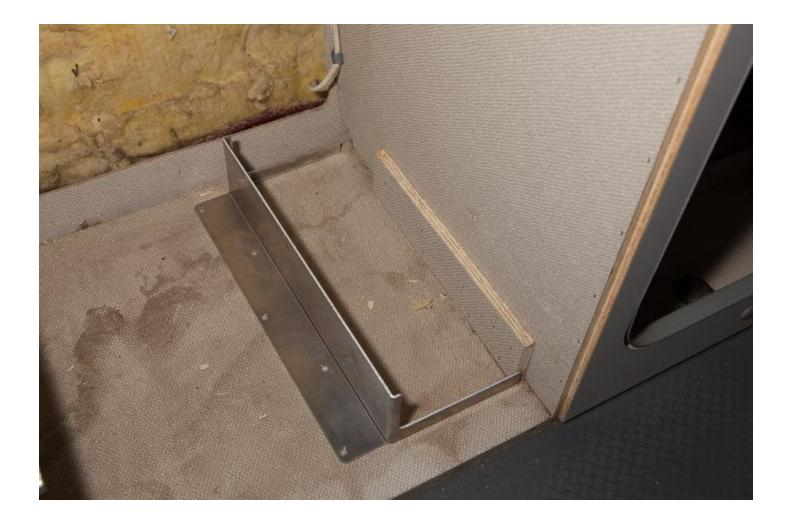
Use a **Drill**, **Drill Bit Extension** and a **Phillips Head Drill Bit** in order to secure five **1/2**" **LG Self Tapping Screws** that are in **Hardware Package B** into the right side of the cabinet wall. This will secure the **Support Bracket** in place.
