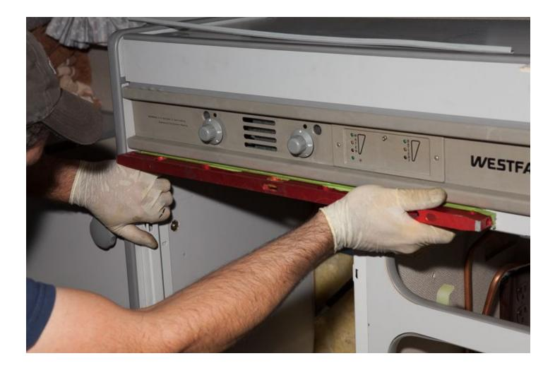
Insert the included **T-Moulding** in the gap in between the stock cabinet face and the newly installed **Side Support Mounting Plate.** This moulding should simply be pressed in by hand.
