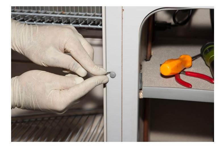
Using a **Phillips Screwdriver**, remove the 5 screws from the face of the stock fridge surround frame.
